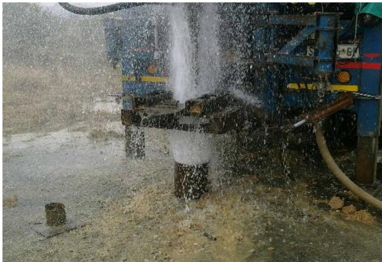
**Figure 3-Typical blow yields during borehole development**
