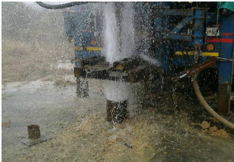
Figure 3-Typical blow yields during borehole development
