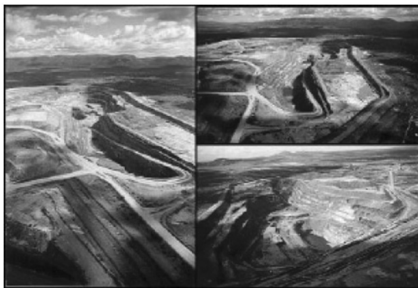
Figure 2. PPRust's Sandsloot open pit
