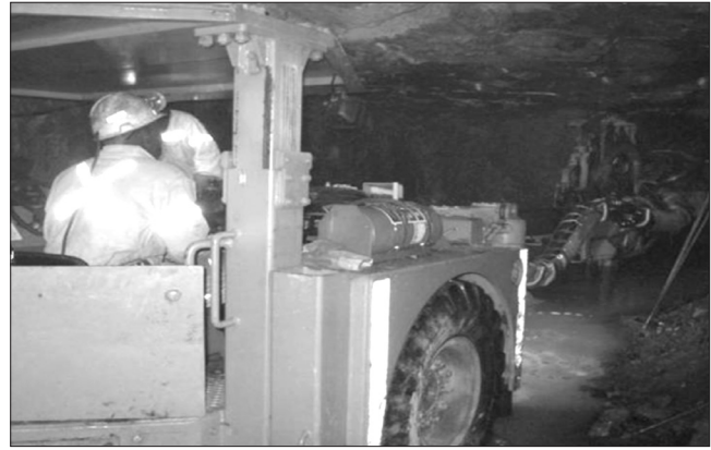
Figure 6. Axsess development rig (face drilling and bolting)
