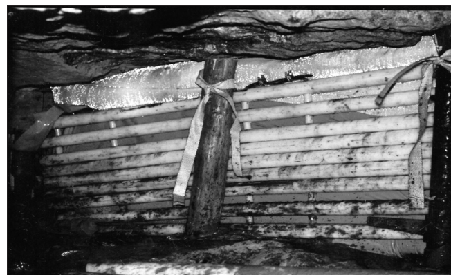
Figure 4. Backfill bag 24 hours after placing of backfill
